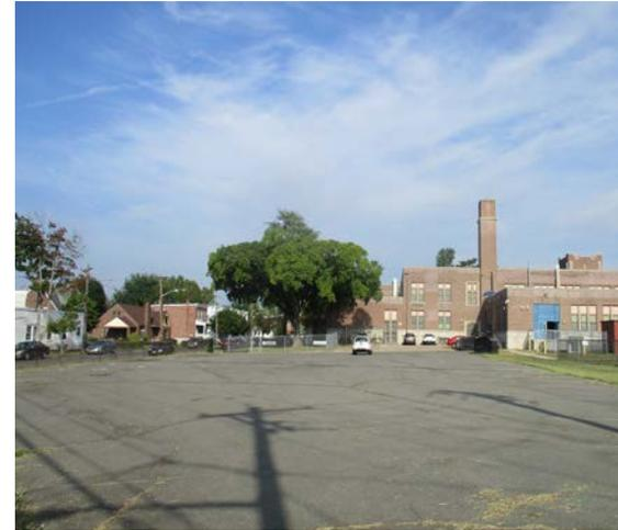
Roof runoff can be captured by installing rain gardens adjacent to the building. Rain gardens can capture, treat, and infiltrate stormwater runoff. The parking lot in the rear of the building is in poor condition. The lot can be converted to porous asphalt to capture and treat stormwater runoff. A preliminary soil assessment suggests that more soil testing would be required before determining the soil's suitability for green infrastructure.
